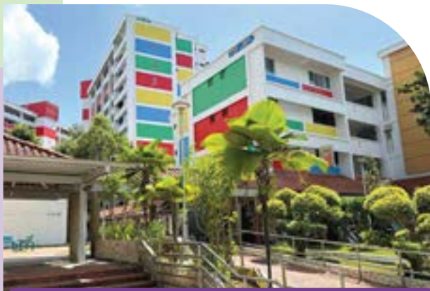
Repainted HDB Blocks from Blks 731 to 735
