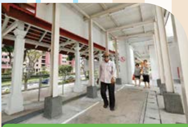
Construction of Shelter over Existing BFA Ramp between Blks 224 & 225
