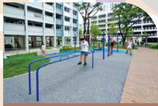
Construction of Fitness Corner between Blks 433 & 435
