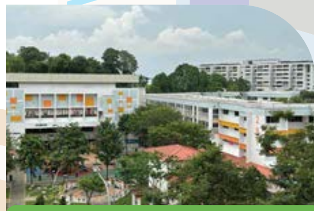
Repainted HDB Blocks from Blks 290 to 294
