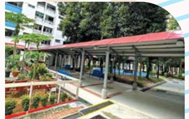
Construction of Low Linkway between Blks 873 & 874
