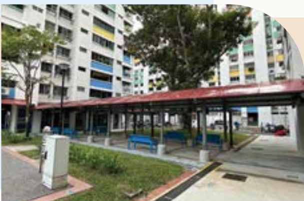
Construction of Low Linkway between Blks 865 & 866
