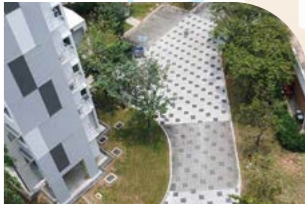
Replacement of Interlocking Tiles at Blks 430A & 430B
