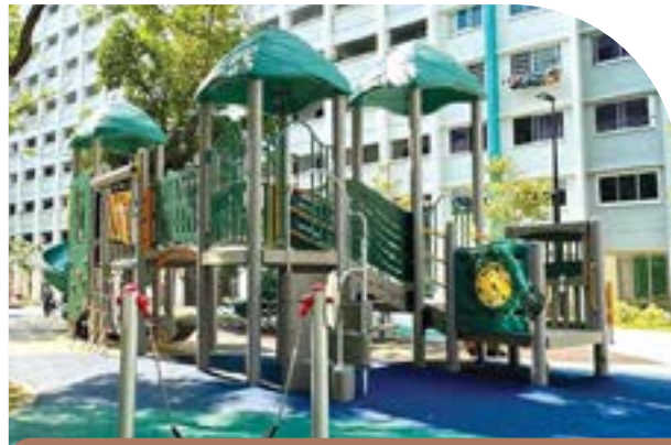
Construction of Playground between Blks 423 & 425
