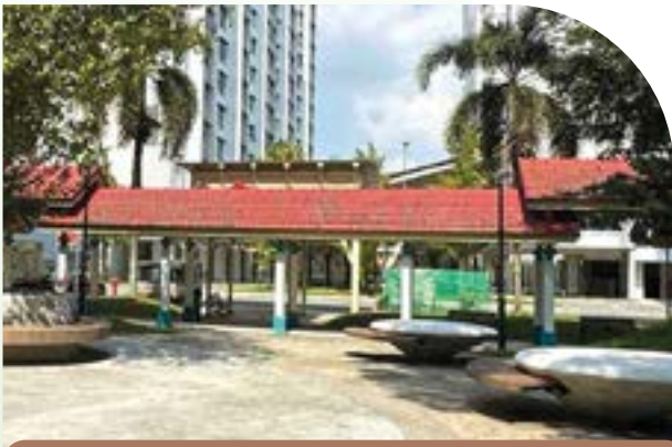
Construction of Footpaths between Blks 423 & 425
