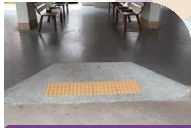
Construction of Ramps at Blks 721 & 782
