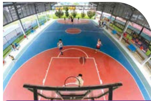
Construction of Sheltered Basketball Court at Blk 761
