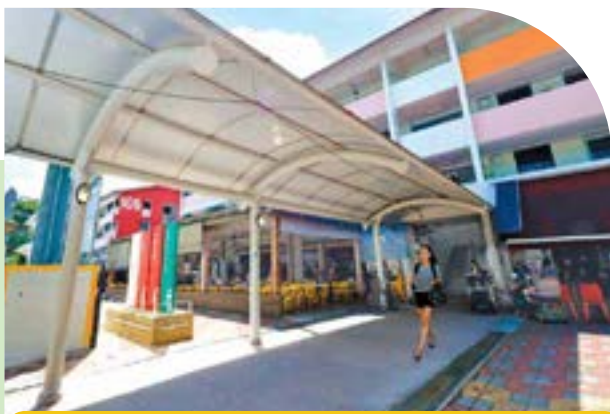
Upgraded Linkway to Coffeeshop & Bus Stop at Blk 101
