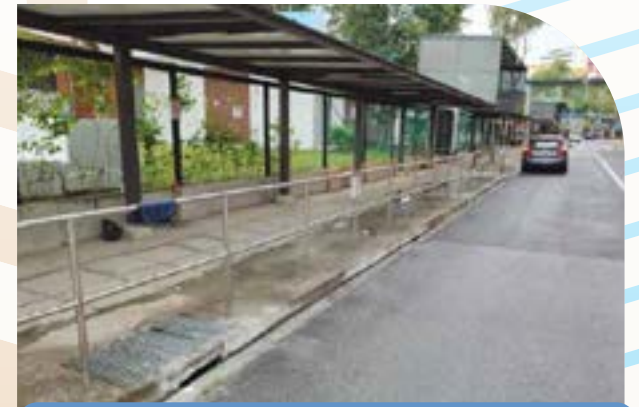
Installation of Railings near Blk 805 outside Peiying Primary School
