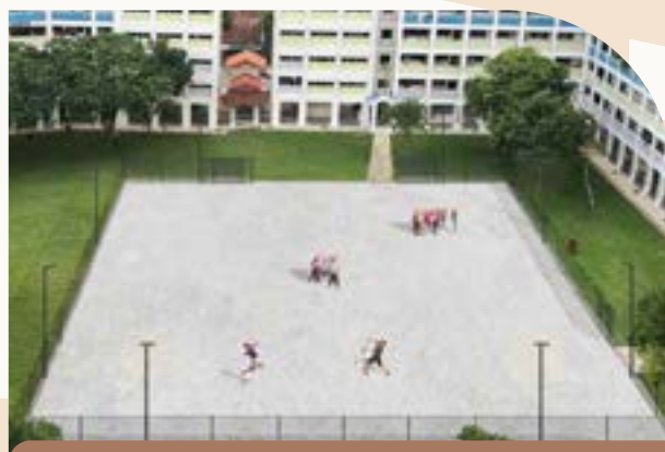
Construction of Hardcourt near Blks 412 & 413
