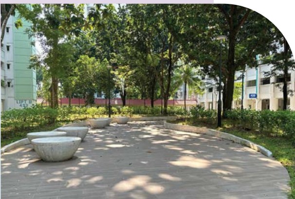
Construction of Seating Areas at Blks 433 to 435
