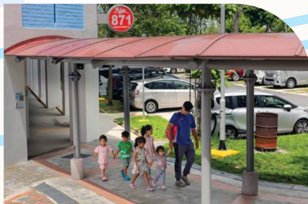
Construction of Low Linkway at Blk 871
