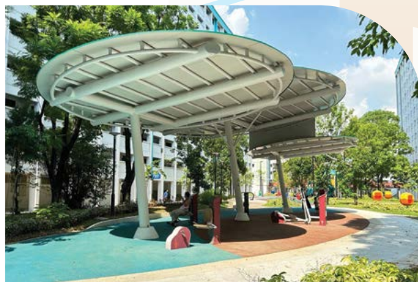
Construction of Sheltered Fitness Corner between Blks 423 & 425
