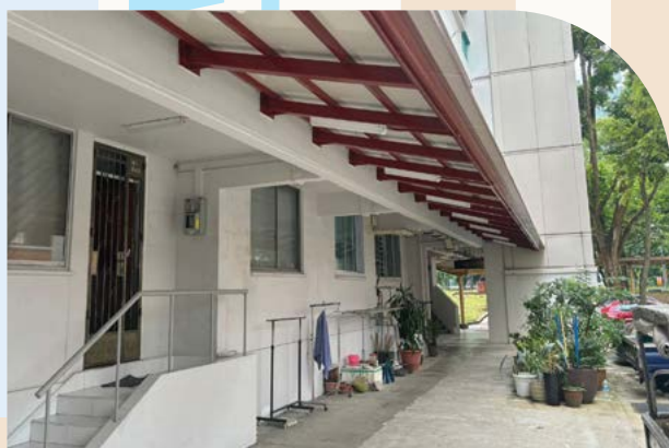
Construction of Awnings at Blks 165 & 175
