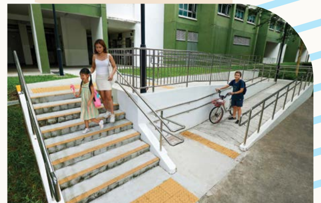
Construction of Staircase and Ramp at Blk 511A
