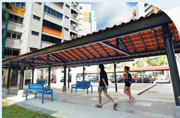
Construction of Low Linkway at Blk 853
