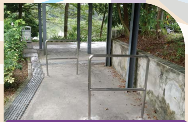
Construction of Railing behind Khoo Teck Puat Hospital
