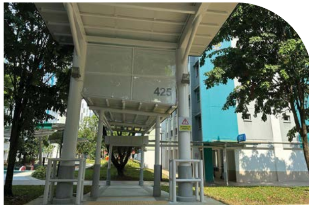
Construction of Linkway between Blks 423 & 425
