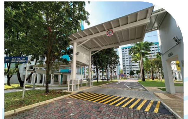
Construction of Linkway between Blks 425 & 428A
