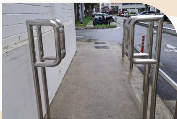
Construction of P Gate Railing at Blk 647
