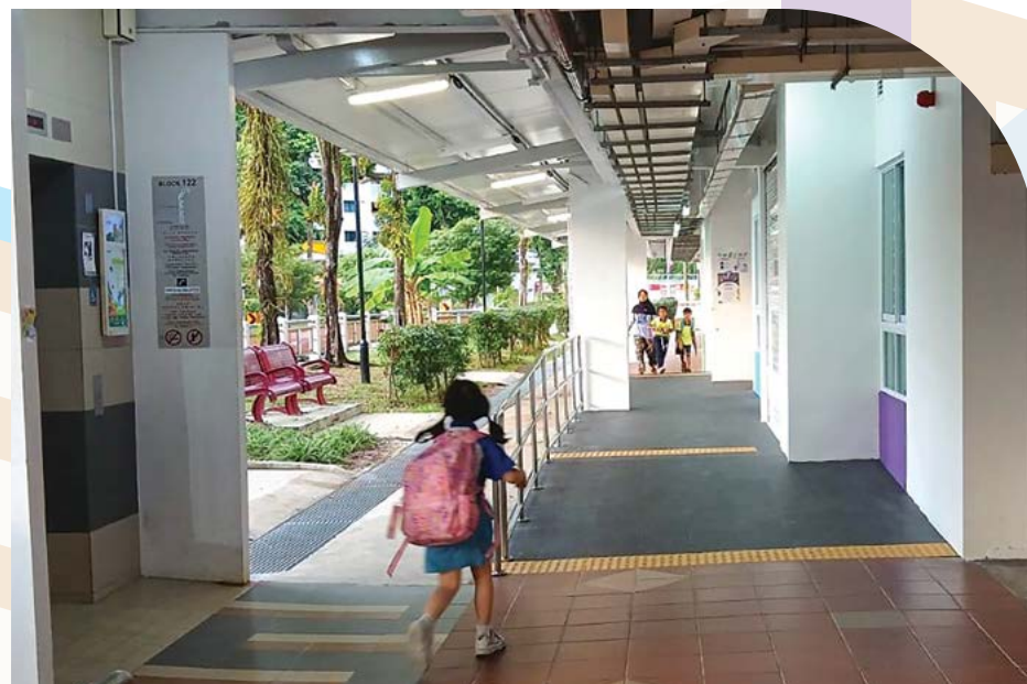
Construction of Awning at Blk 122
