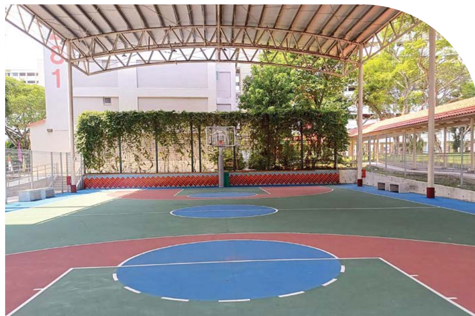
Construction of Sheltered Basketball Court between Blks 281 & 282
