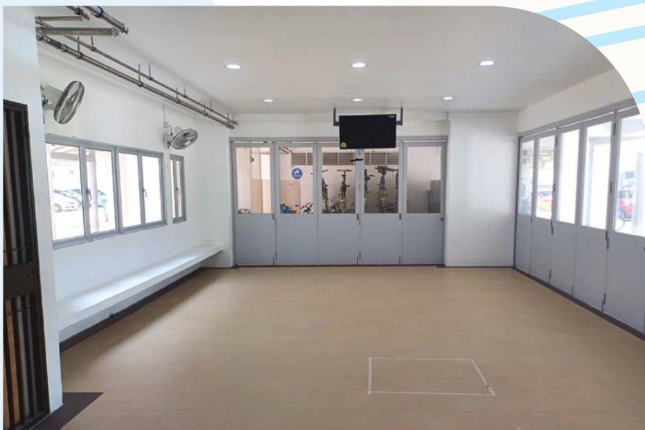
Construction of RC Centre at Blk 287
