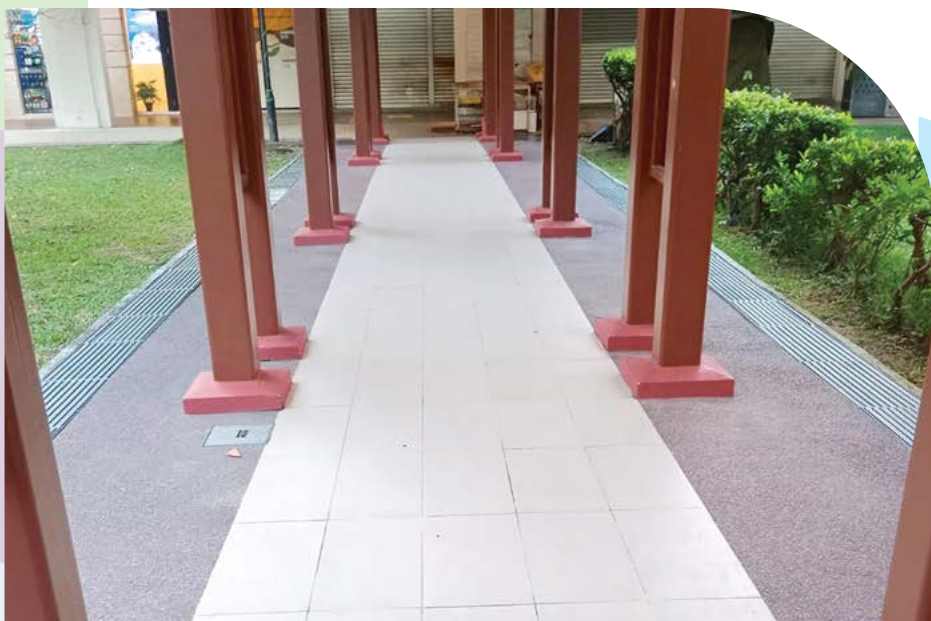
Application of Anti-Slippery Solution to Sheltered Walkway at Blk 850
